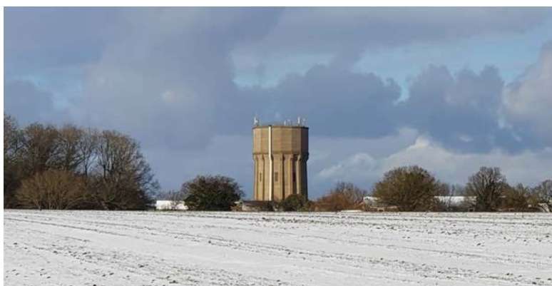
Figure 42: The Water Tower, Rendham Road.
