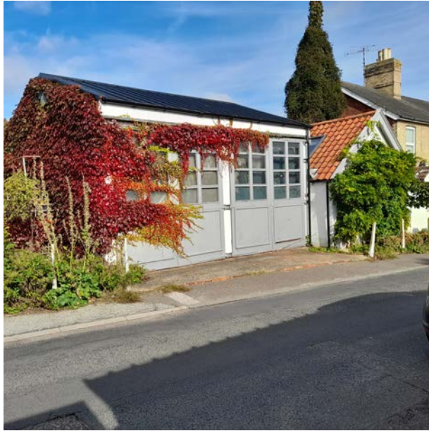
Figure 34: The Old Fire Station, Rendham Road.
