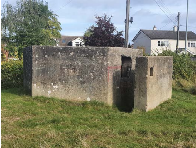
Figure 38: The Pill Box on the Memorial Field.
