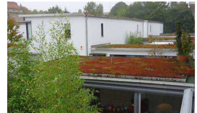
μ Fig. 6.15 Example of green roofs
